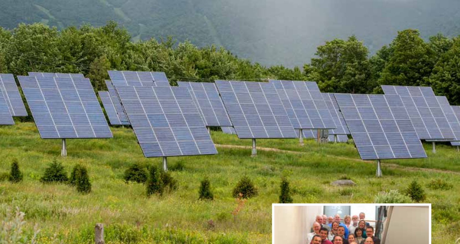
Solar panels provide an alternative form of electricity.
